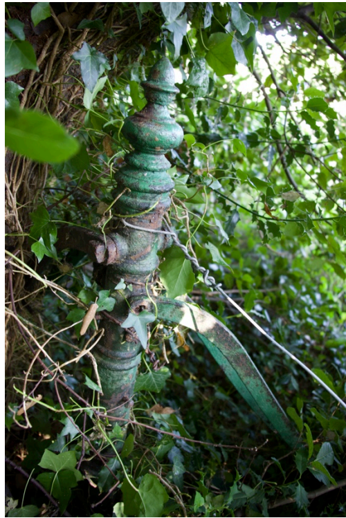
Figure 8.2 Stanchions for the wire fence, the stay resists the tension in the wire fence. The stanchion on the right is a corner post where the fence changes direction around the granite outcrop. and has stays
